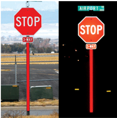
Reflective Tape on Sign Poles
