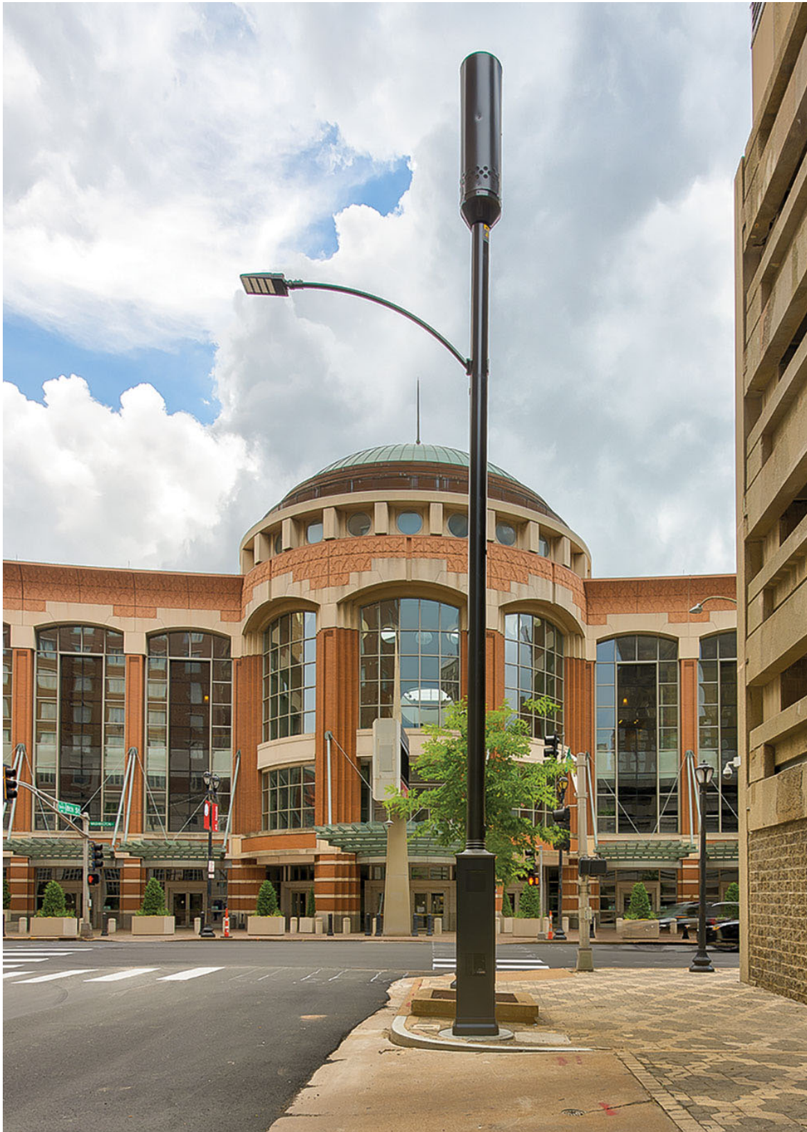
5G Installation Option: A partially concealed small cell topper on a light pole in St. Louis. Photo by Raycap.
