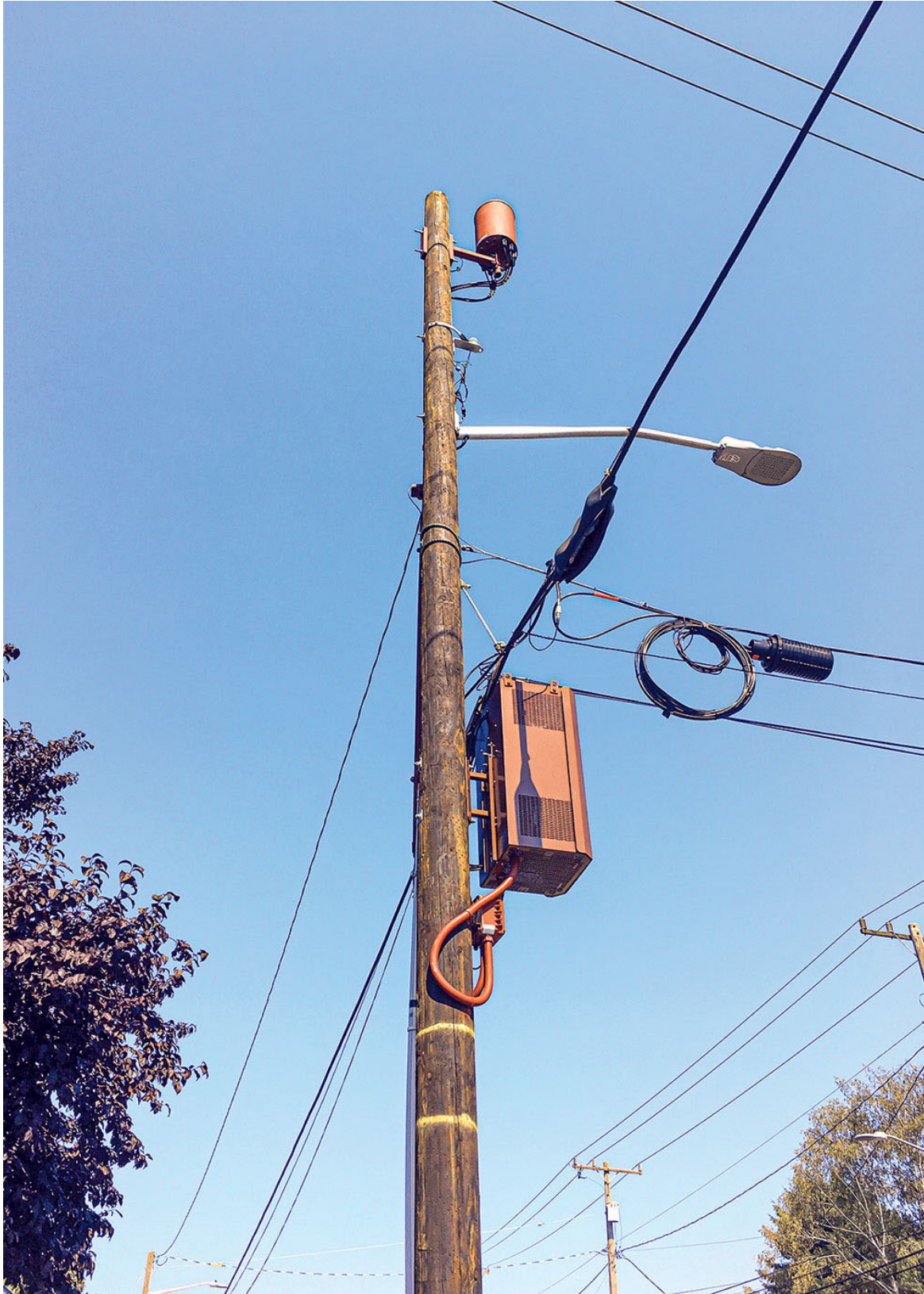
5G Installation Option: Mounted on a combination lamp post and telephone pole in Seattle. Photo courtesy Seattle Department of Transportation.
