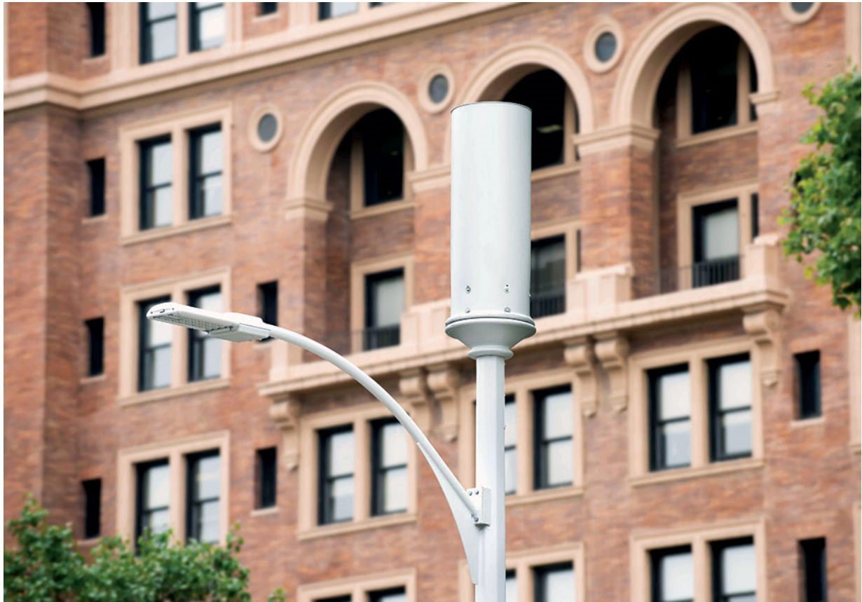
A small cell on a light post in Pittsburgh. Photo courtesy Crown Castle.
