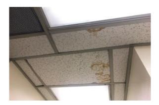
Wall coverings, ceiling tiles, floor coverings, and wall and ceiling insulation should be inspected to identify the presence of damage or mold growth. Both exposed and concealed surfaces should be inspected.
