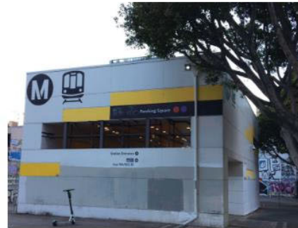
Constructed above is a wooden box over the entrance portal for overhead protection at the 4th/Hill Station.
