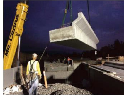
Overhead protection is required when moving heavy objects over Metro ROW or in areas designated for public use.
