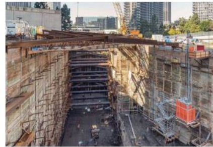
Excavation and shoring plans must be reviewed by Metro to ensure structural compatibility with Metro infrastructure and safety during adjacent development construction.
